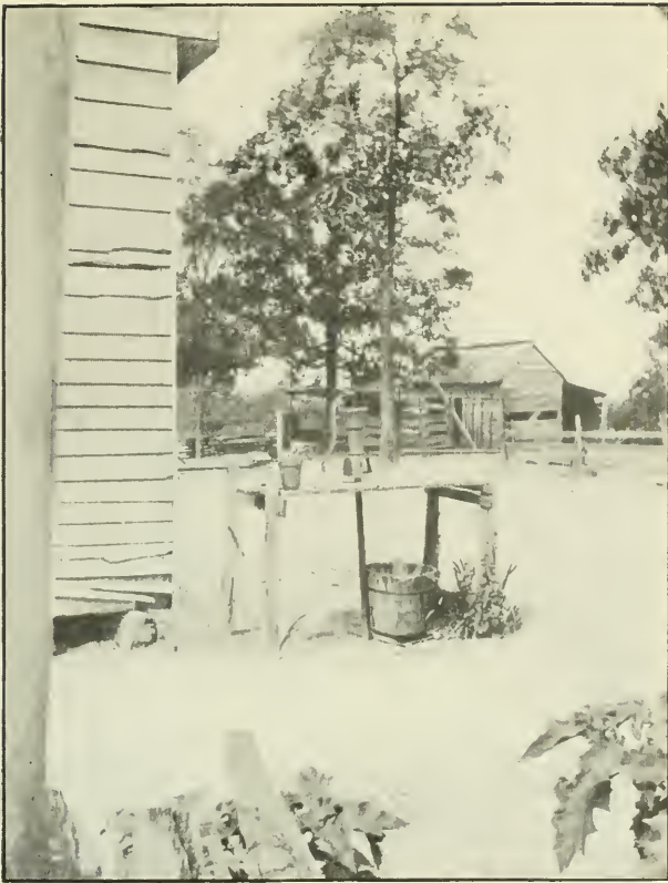
PLATE XII.—DRILLED WELL CONVENIENTLY NEAR THE HOUSE.
